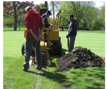
Vibratory plows cut slots in the soil rather than digging a trench to minimize turf damage
